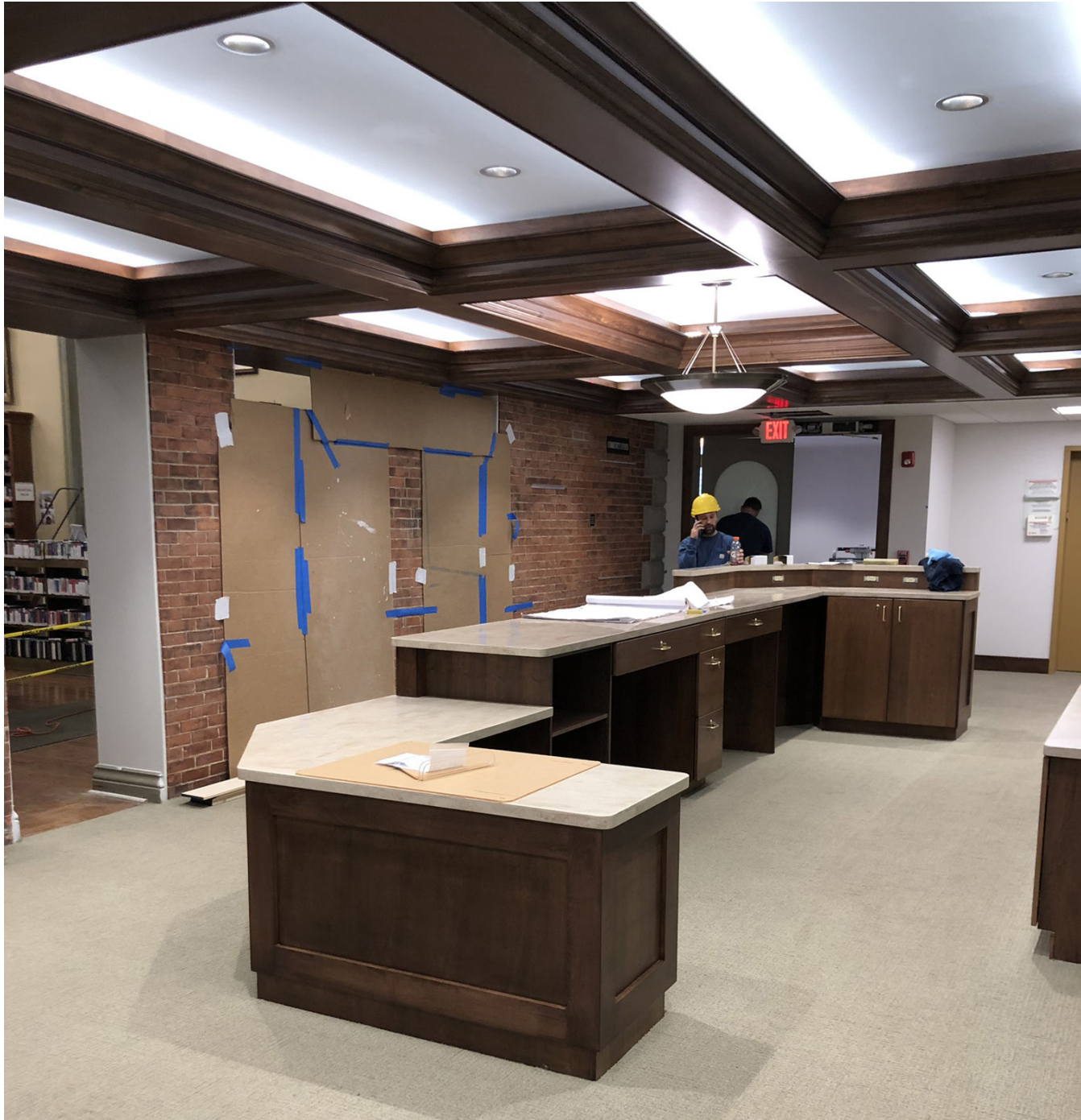
Circulation area in progress
