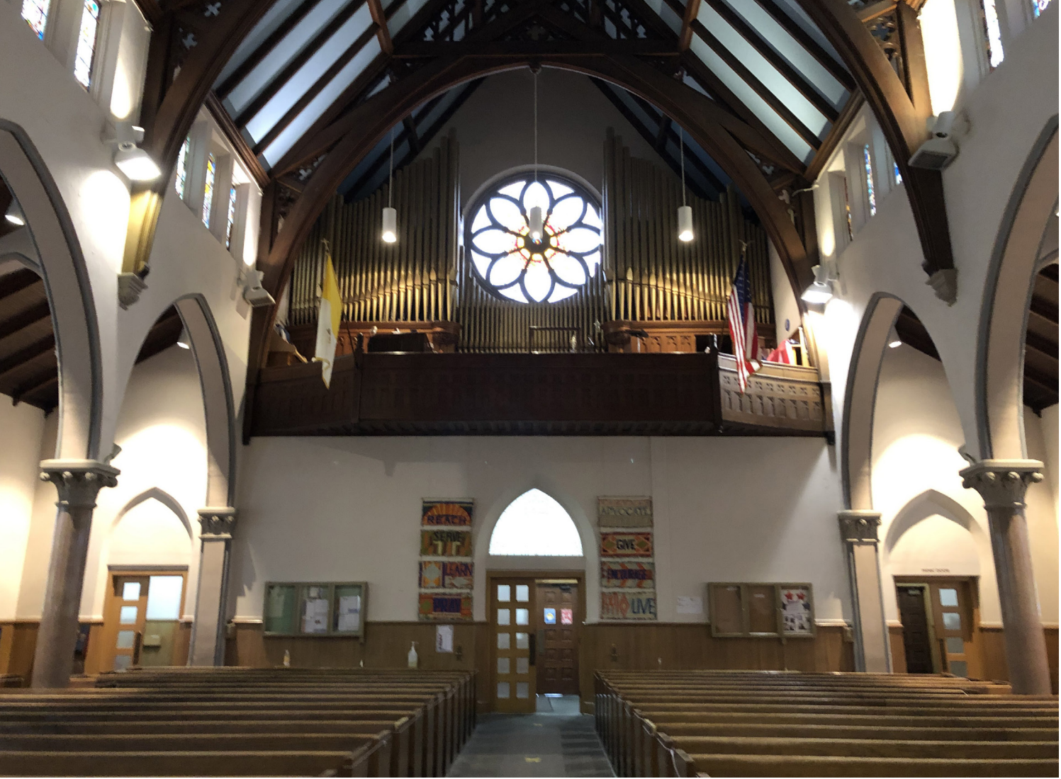
Existing rear Nave
