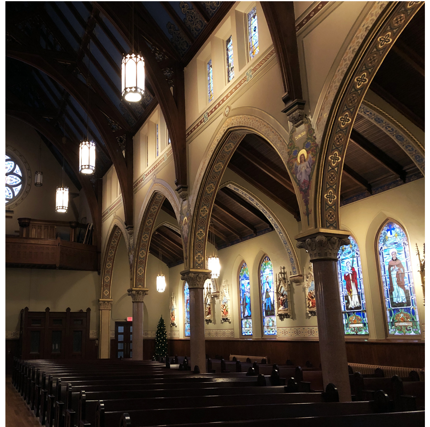
Side aisle view, after
