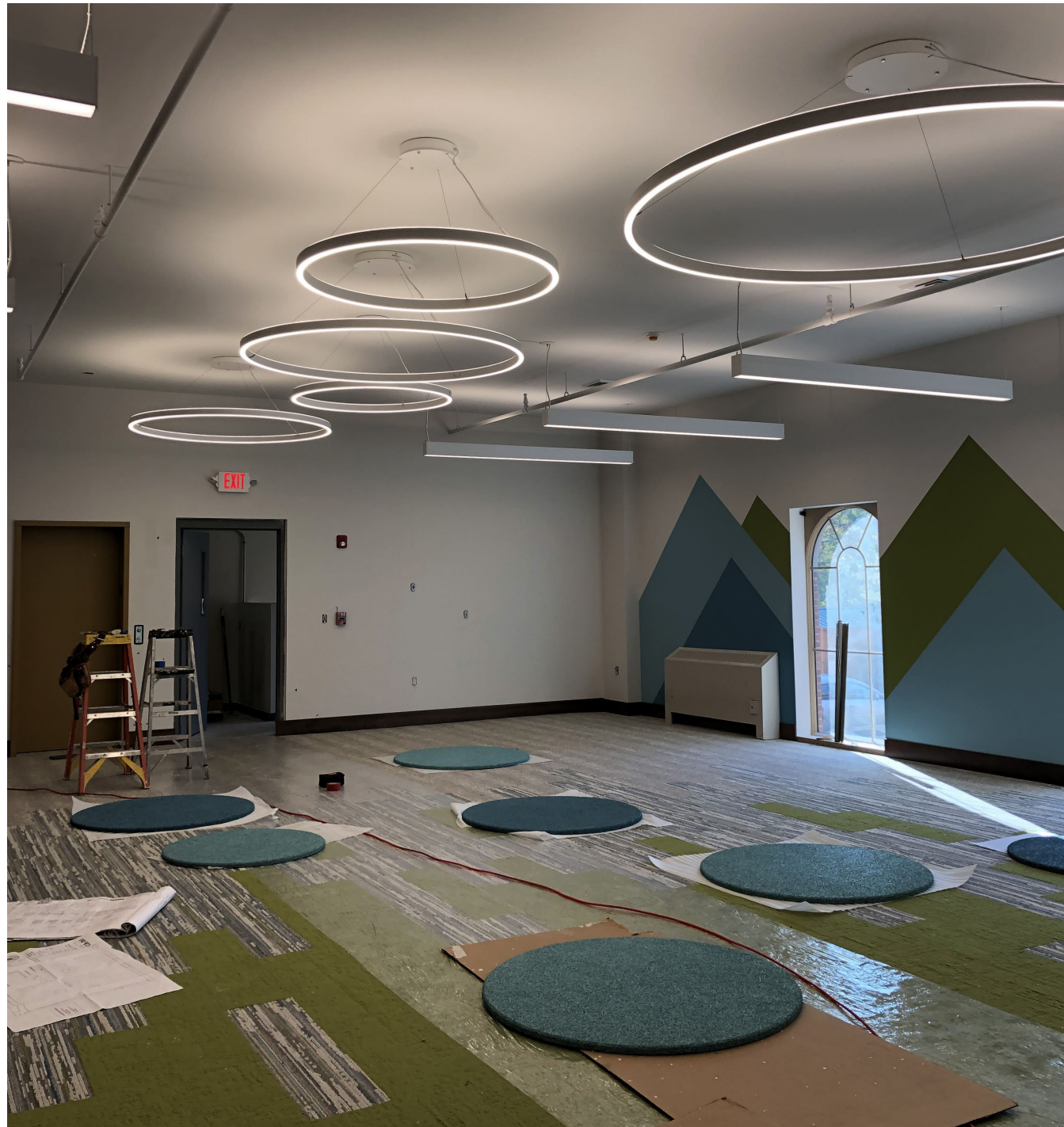
Children's library in progress
