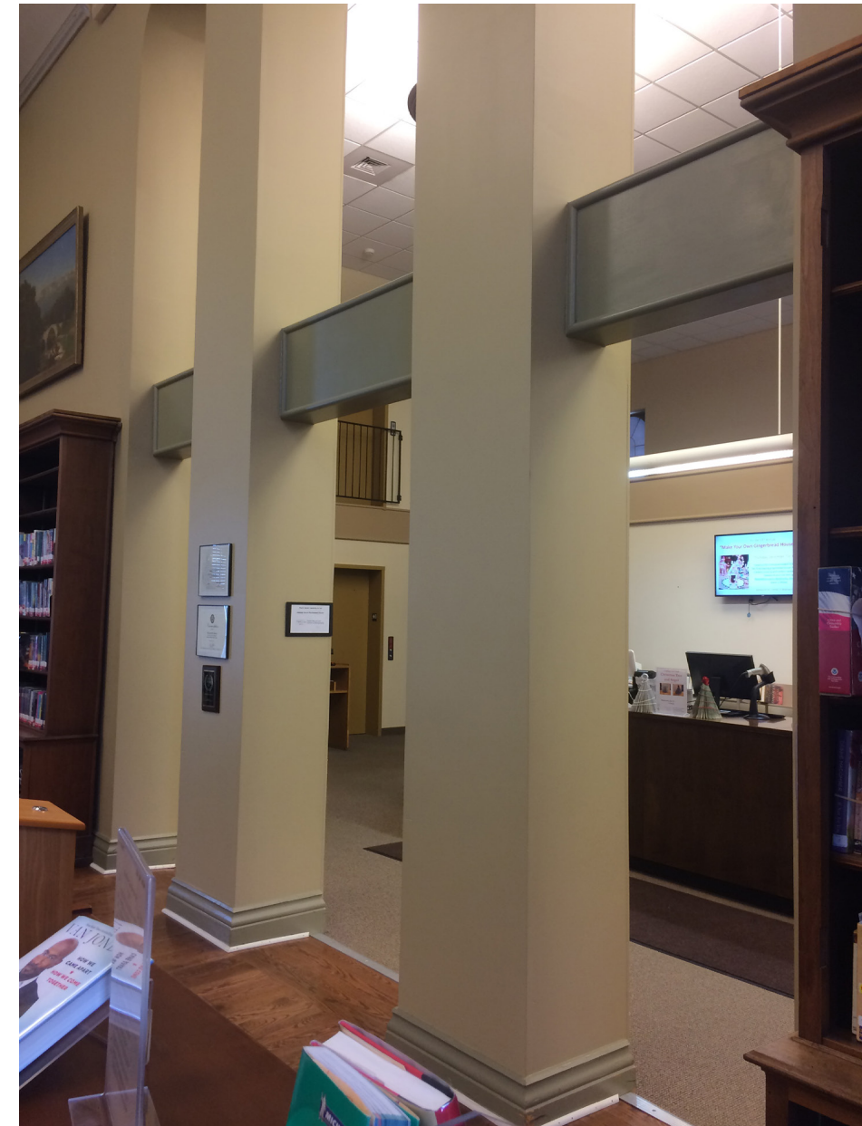
Existing circulation room view
