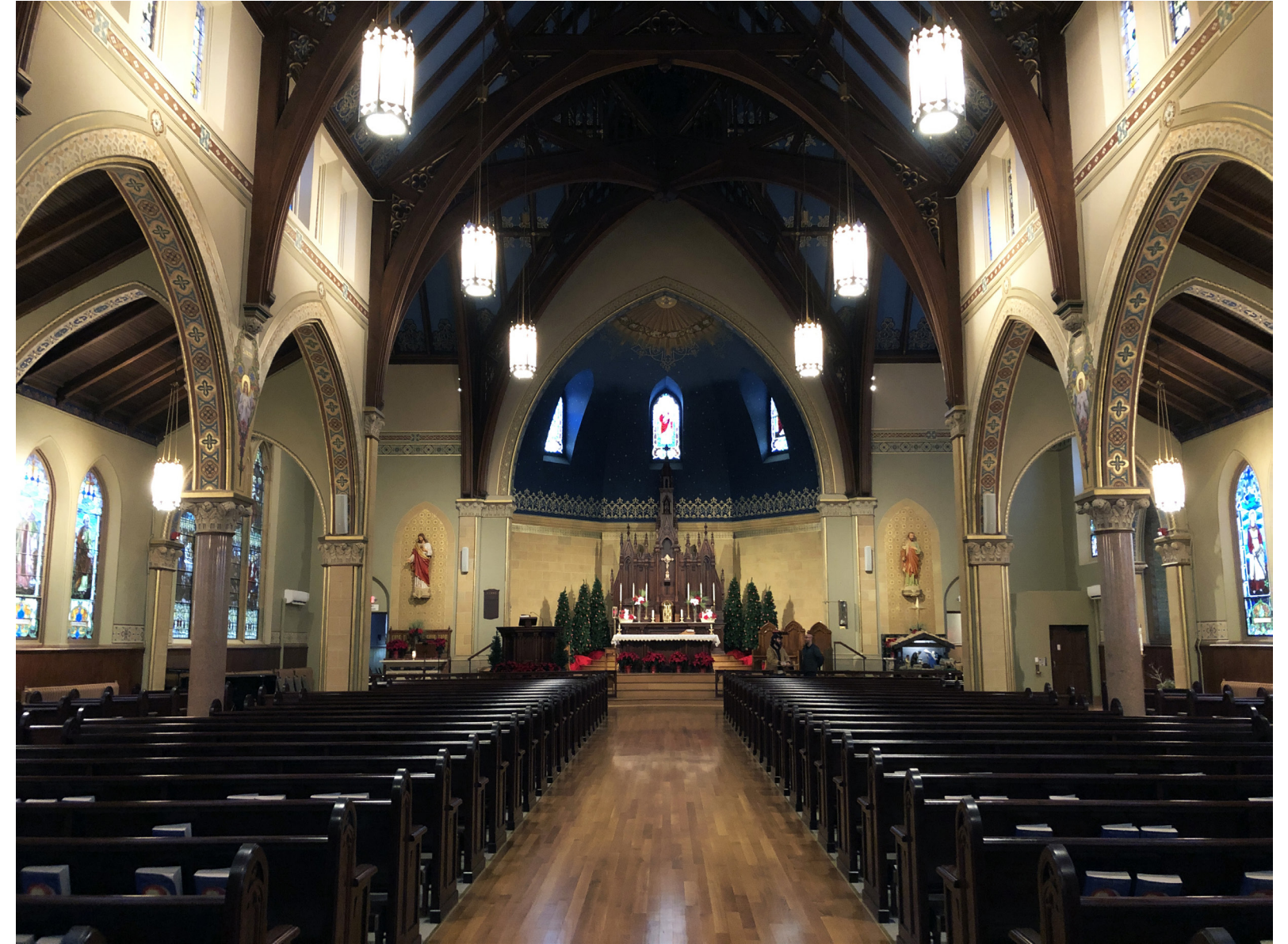
Sanctuary view, after
