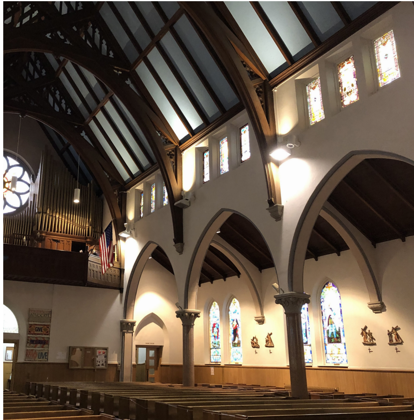
Side aisle view, before
